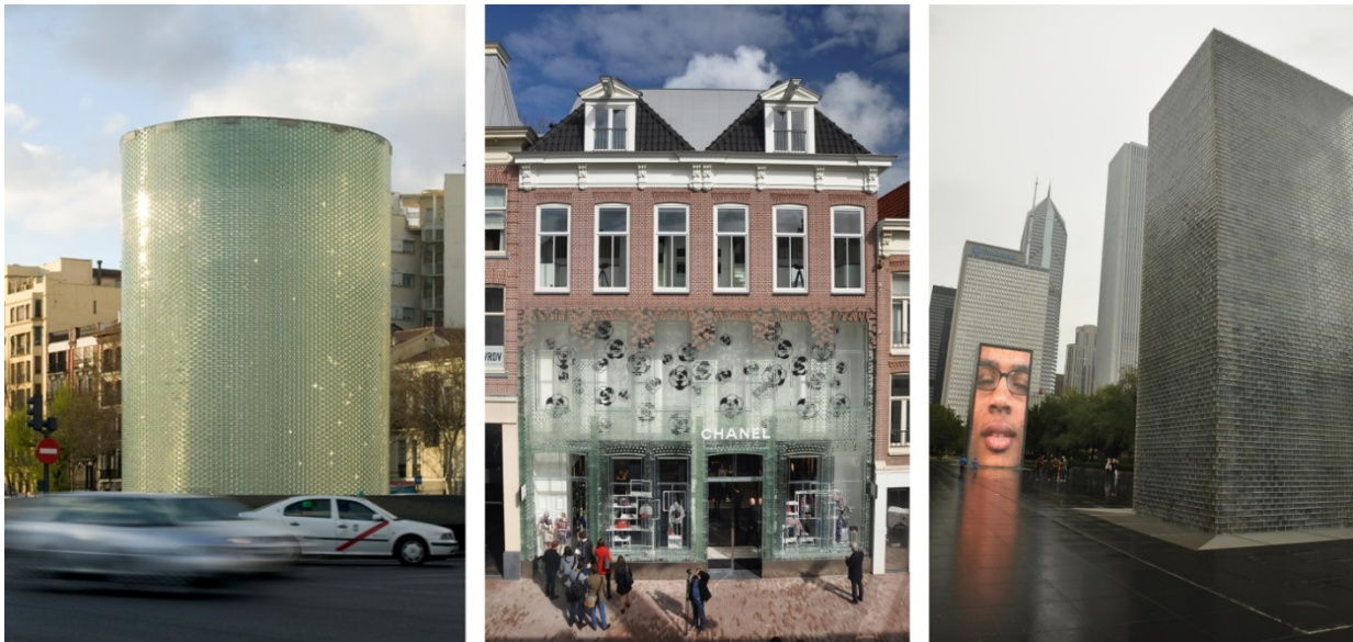
Fig. 1: Some of the most characteristic examples of structures out of cast glass blocks: The adhesively bonded Atocha Memorial (left) and Crystal Houses (centre), and the Crown Fountain (right) which is supported by a metal substructure.
