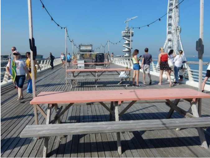
Figure 70: View of the top floor of the pier.
