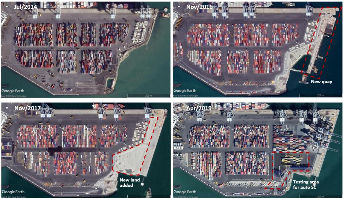
Figure 5-7: implementation process of new auto SC of Fergusson terminal, port of Auckland, New Zealand.
