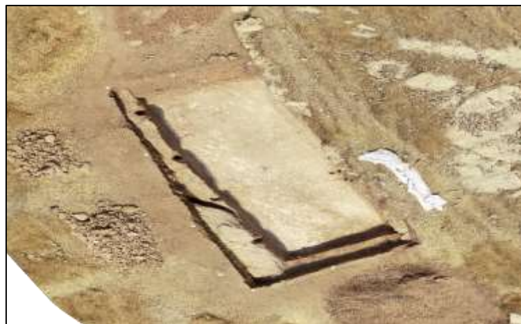
Figure 5 An example part of the Faida canal exhibiting a rectangular cross-section, by the LoNAP team.
