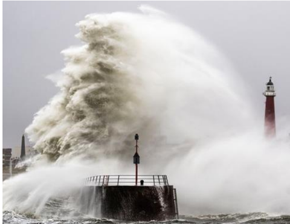
Figure 1 Wave overtopping event at a breakwater affected by wind.
