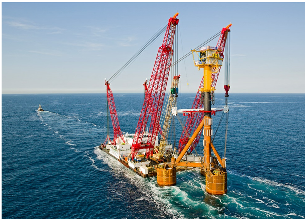
Figure 8.5: A heavy lifting vessel [Scaldis Salvage Marine contractors NV, 2019]
