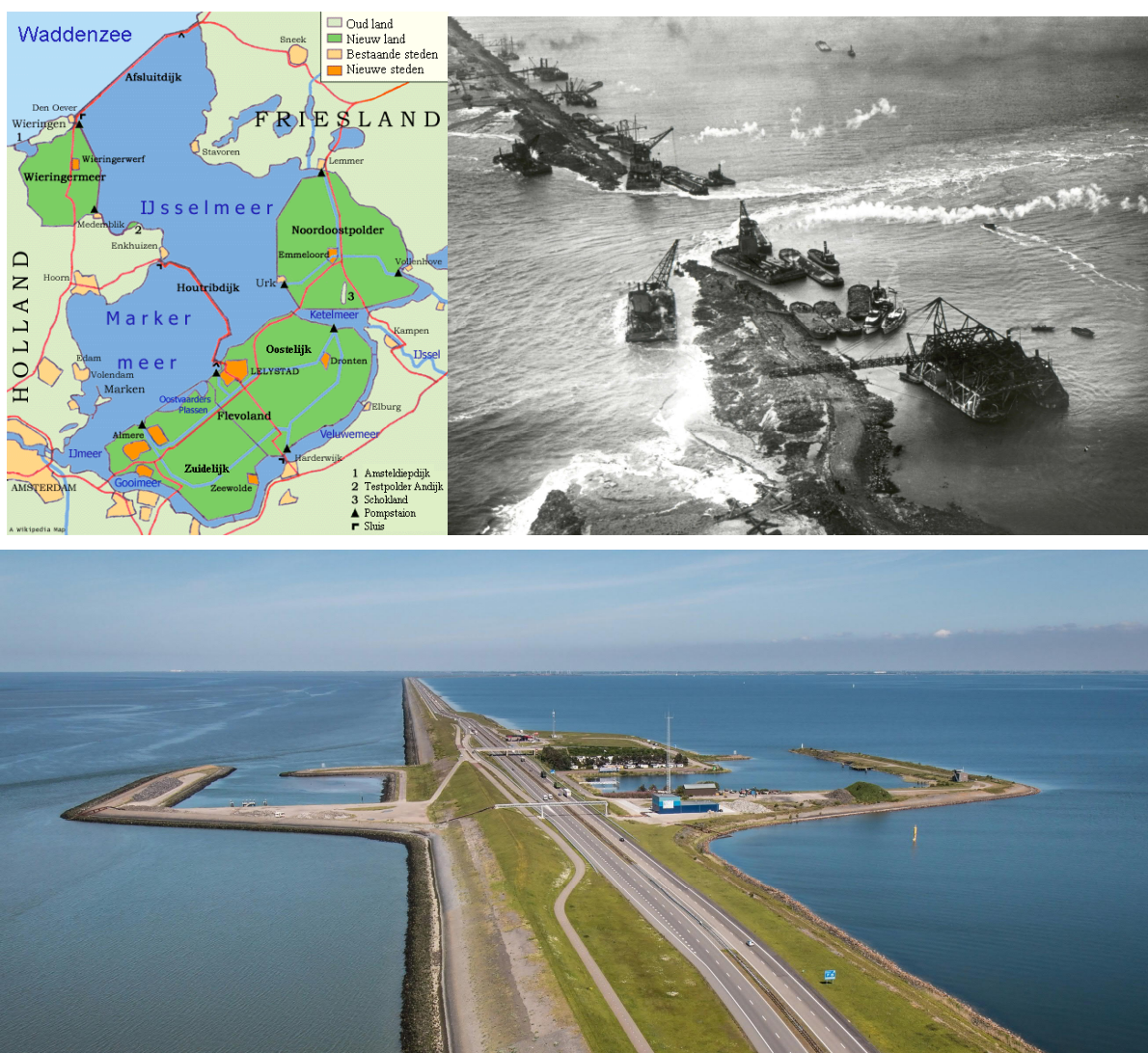
Figure 1. Illustrations of Afsluitdijk, top left: location, top right: closure during construction in 1932, bottom: recent photo of the dam at location Breezanddijk (courtesy: Rijkswaterstaat beeldenbank)
