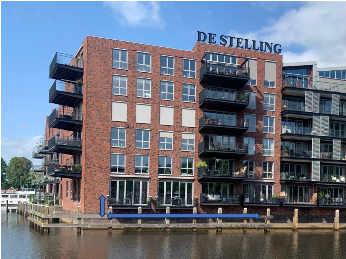
Figure 35: Construction in Kraanbolwerk, Zwolle (Photo by author)
