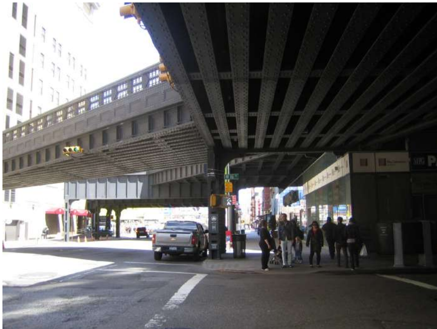
Fig. 26. A trait of the High Line seen from an unusual perspective. Safety issues have to be addressed with more care in these under-structure “blind spots”.
