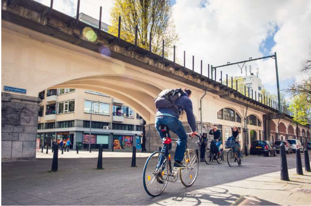
Fig. 32. The Hofbogen viaduct south of Bergweg Station.
