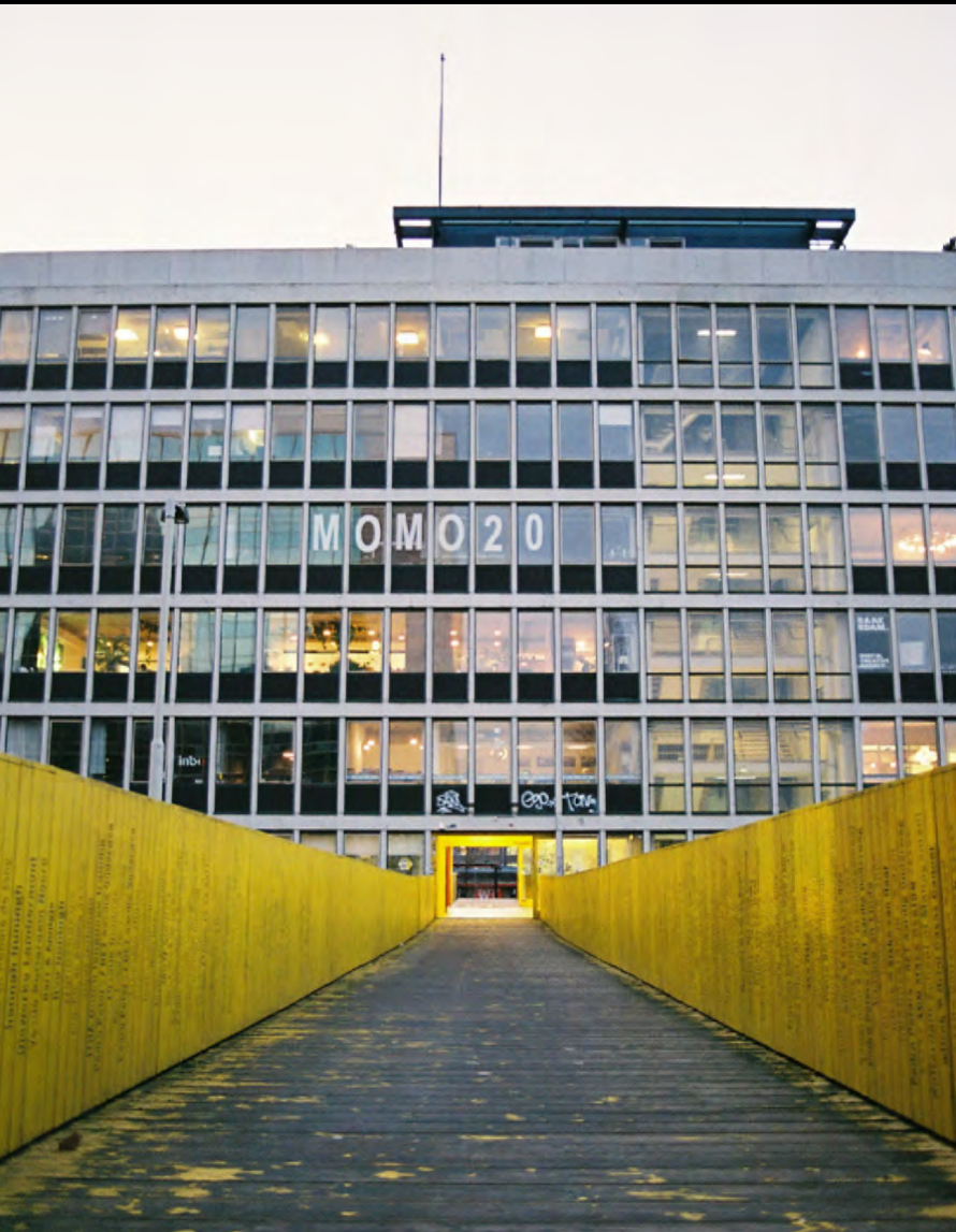
Figure 65: View on Schieblock from Luchtsingel
