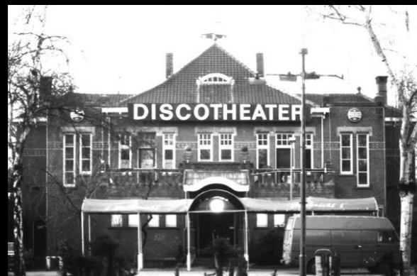
Figure 11: Former club Parkzicht in Het Park in the 90s (XXL Radio, 2023)
