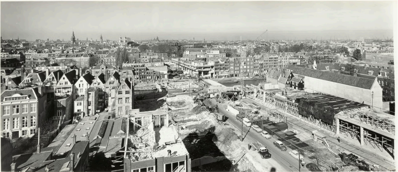
[04] the Weesperstraat during urban renewal in Amsterdam
