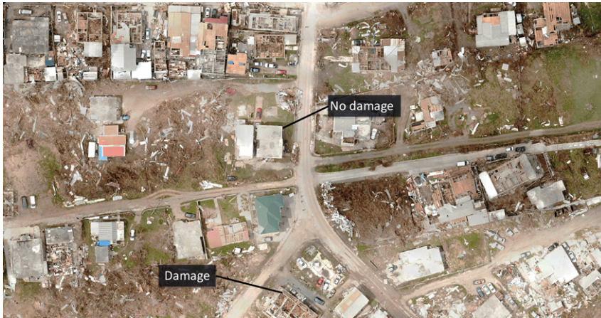
Figure 2.2: Example of damage detection [Based on: Netherlands Red Cross (11 Sept. 2017), Cole Bay - Sint Maarten [georeferenced image], used under CC-BY4.0 as part of Open Imagery Network, retrieved from www.openaerialmap.org ]
