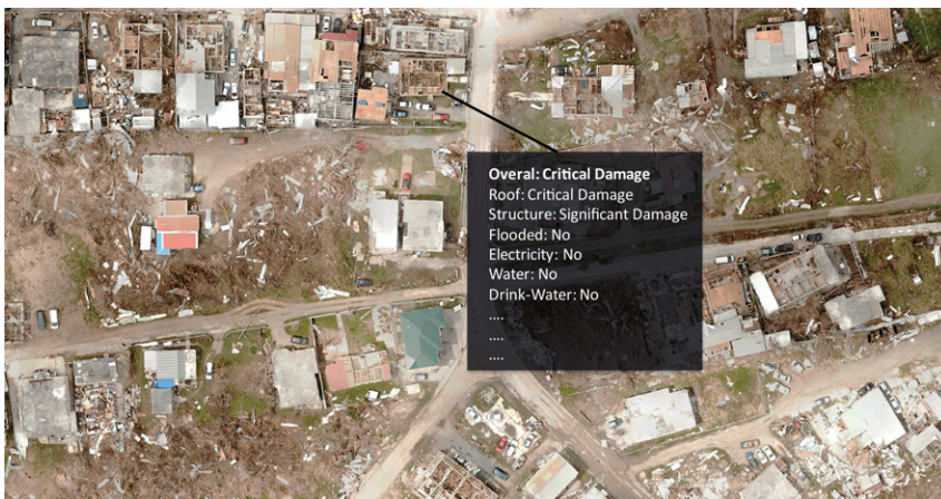
Figure 2.4: Example of damage assessment [Based on: Netherlands Red Cross (11 Sept. 2017), Cole Bay - Sint Maarten [georeferenced image], used under CC-BY4.0 as part of Open Imagery Network, retrieved from www.openaerialmap.org ]
