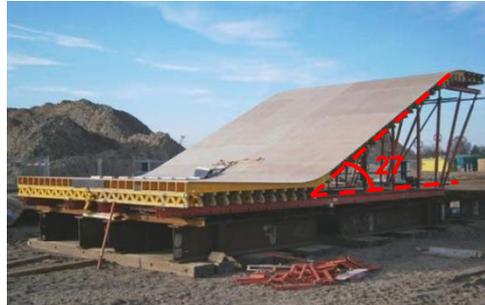
Figure 7.1. Concrete formwork sloped at 27 degrees for the “Promenadebrug Nijmegen, the Netherlands (2015). Photo: *Betoniek* 2015-12
