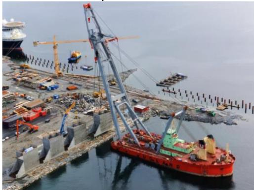
Figure A.23. Vestbase Kai, caissons lifted by a 800 tonnes floating crane (2010), Uglund Marine Services AS, HLV UGLEN<sup>17</sup>
