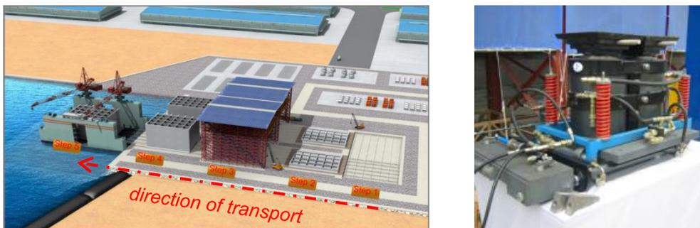
Figure 4.9. Caisson transport and launching; 5 phase transport to floating dock (left) and 250 tonne jack (right) (Bygging-Uddemann 2017)
