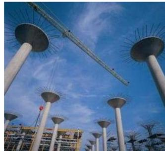
Figure 1.7. Multiple cone shaped column heads
