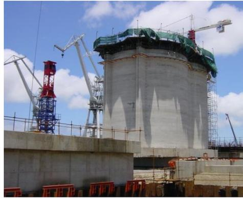
Figure A.5. Traditional slipforming used for one of the caissons
