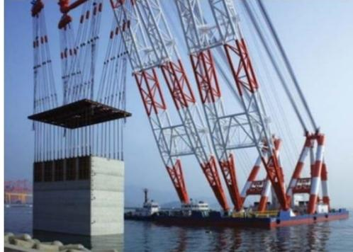
Figure A.22. Prestressed caissons lifted by a 4,000 tonne crane (Port of Busan, Korea, 2008)<sup>16</sup>
