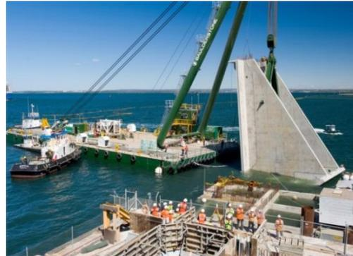
Figure A.25. The 700 tonne shear leg barge lifting a 650 tonne counterfort element
