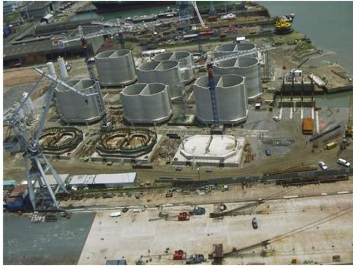
Figure A.4. Bi-circular caisson construction for the Port of Durban (South-Africa, 2004)
