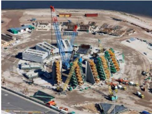
Figure A.24. The 460 tonne ringer crane and counterfort elements
