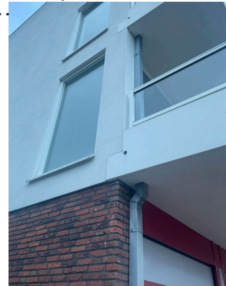
Pipes on the facade
