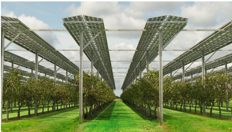
Figure 3.2: Agri-PV orchard consisting of multiple crop strips with the same pitch as the PV array.
