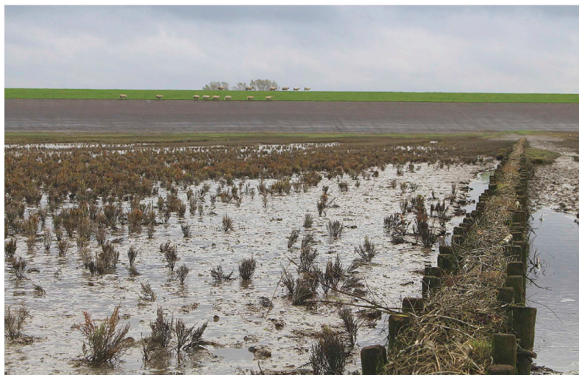
Fig. 3. Brushwood dams in the Dutch Wadden Sea, which create artificial shelter for salt marsh vegetation from waves and currents. The dike is visible in the background (Photo: V. Vuik).
