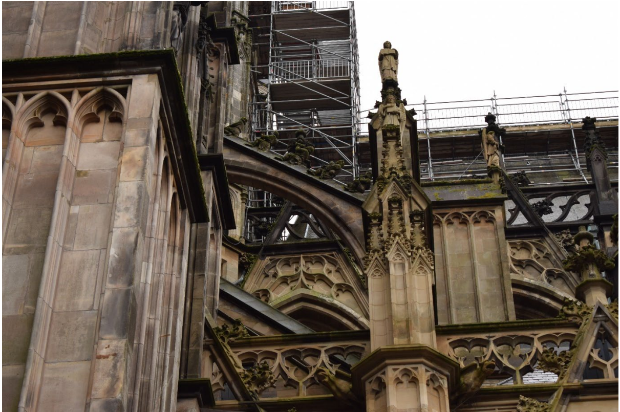
The flying buttresses on the east side of the south transept, with figurines.
