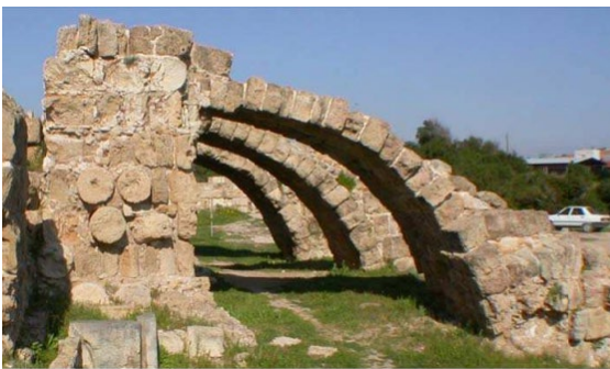
Figure 5: Early flying buttresses in Salamis-Constantia, Byzantine Cyprus 40
