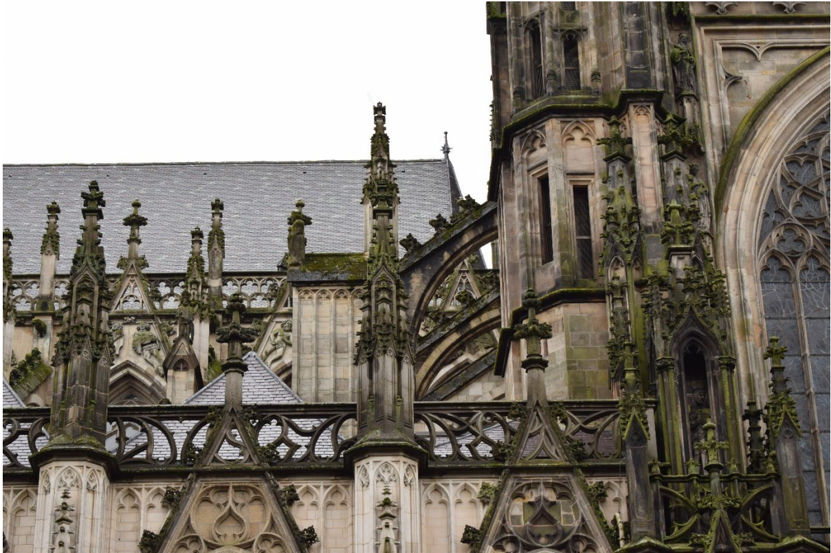
The flying buttresses on the west side of the south transept.
