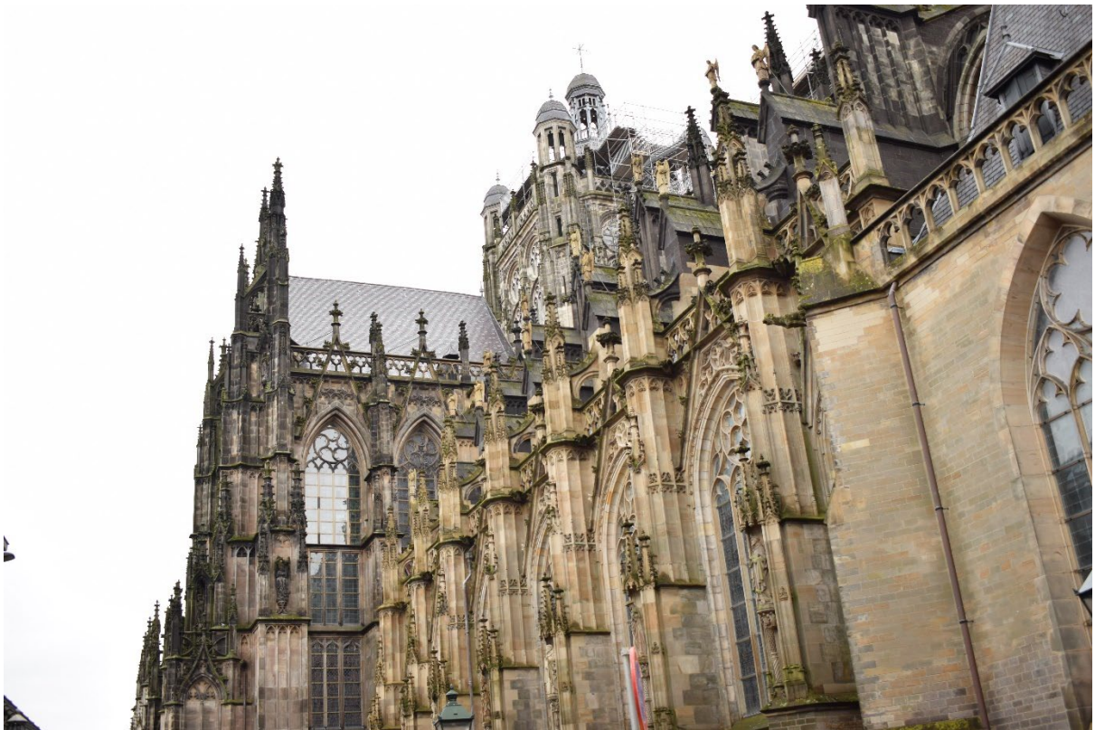
Pier buttresses of the choir.
