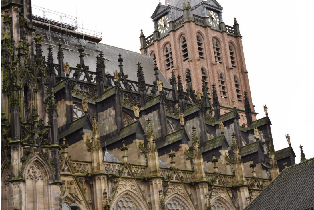
Northside of the Nave with the flying buttresses and flyer chairs.
