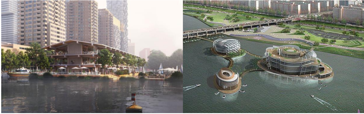
Figure 7 - Floating office Rijnhaven, Rotterdam (left). image: Powerhouse Company. Sebitseom, Floating island on the Han River in Seoul, South Korea (right). Image: Haeahn Architecture.
