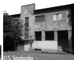
HOUSES FOR EMPLOYEES
