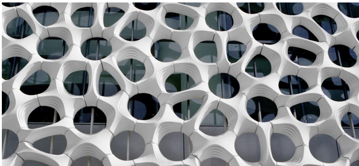
Figure 22 Photocatalytic facade of Torre de Especialidades Hospital Manuel Gea Gonzales, Mexico
