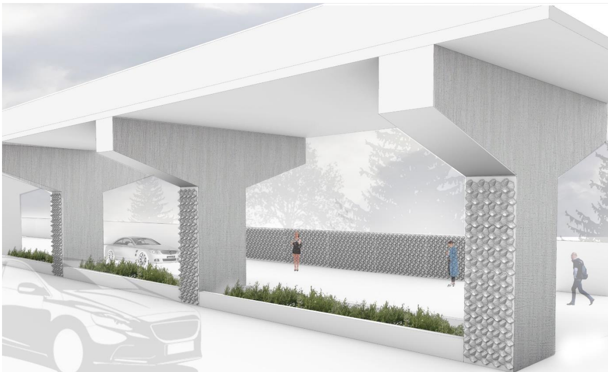
Figure 81 Application of facade panels as acoustic barriers and cladding for elevated roadways
