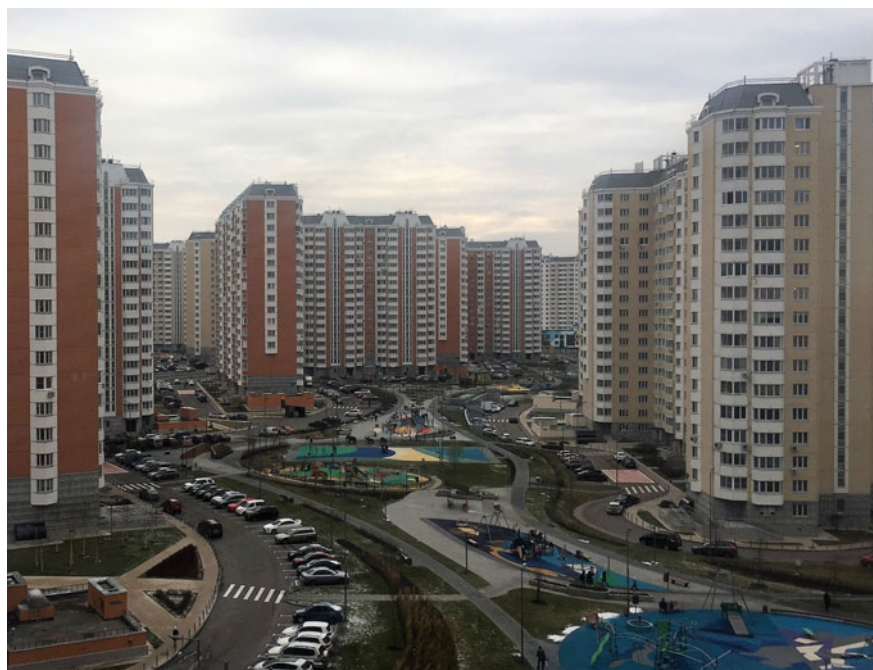
Fig. 13.5 Post-Soviet large housing estate in Vnukovskoe settlement, New Moscow. Source Maria Lazareva
