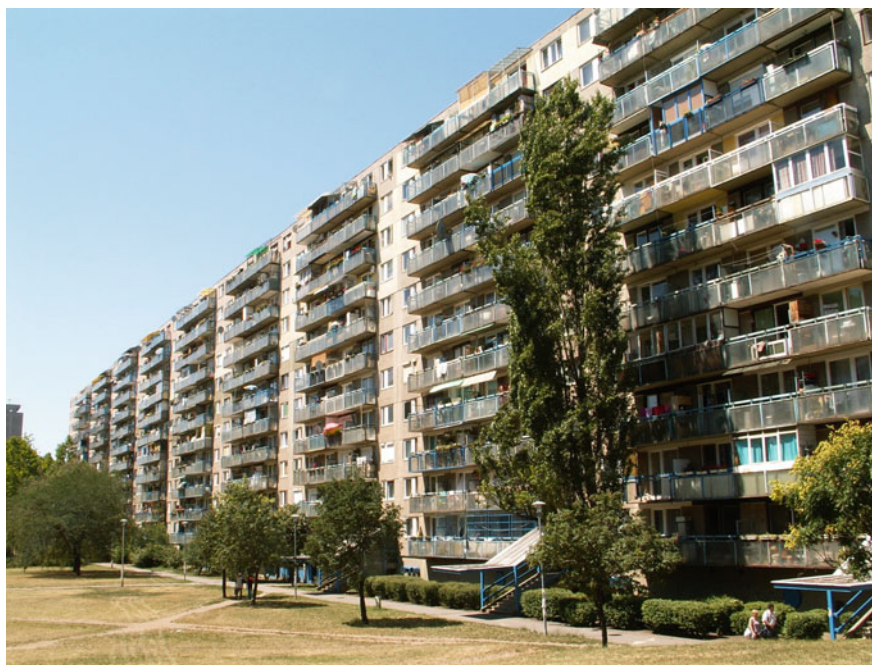
Fig. 9.5 Havana housing estate in the 18th district of Budapest, built using pre-fab technology in the late 1970s. Source Kovács, Egedy and Szabó
