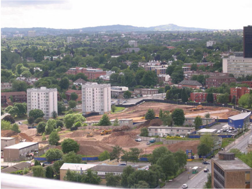
Fig. 6.9 Refurbished tower blocks alongside cleared sites being prepared for new parks and new mixed-tenure housing. Source Birmingham Library Archives and Optima Community Association, used with permission
