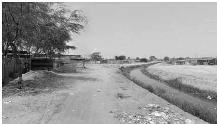
Image 19: Exposed water channels, soft limits Source: Image taken by the author
