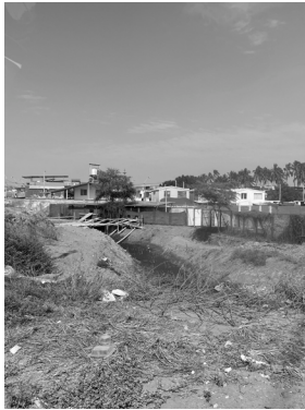
Image 22: Occupation in flood-prone area Source: Image taken by the author
