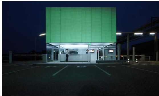
Figure 3. Retro-reflective facade (Musch, 2013)
