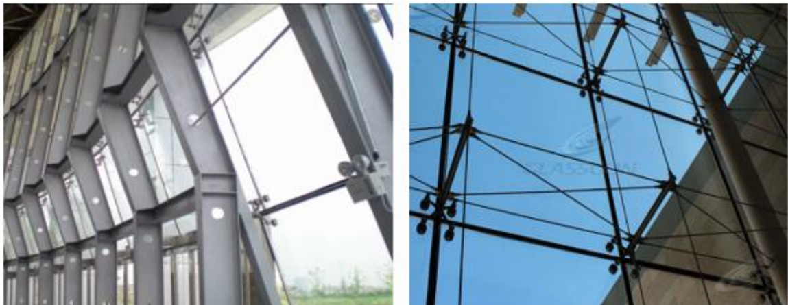
Figure 2: stabilizing and connection of glass façade
