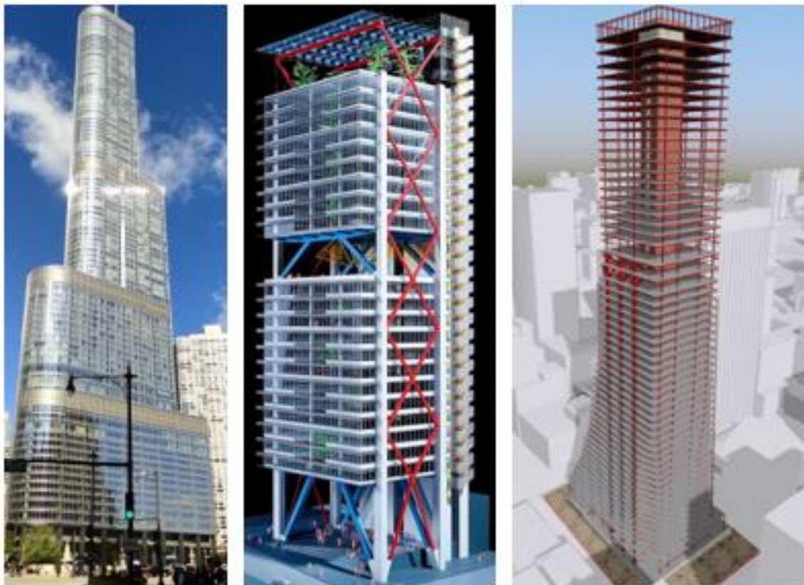
Figure 22: stability of high-rise buildings in concrete, steel, and composite (concrete and steel)
