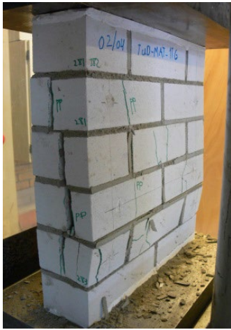
(b) CS brick masonry failure mode
