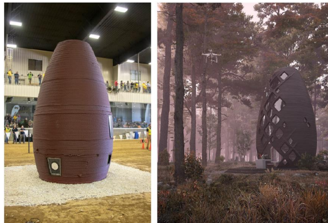
Figure 15. Martia and Tera 3D printed structures by AI Spacefactory Source: (AI Spacefactory, 2020)
