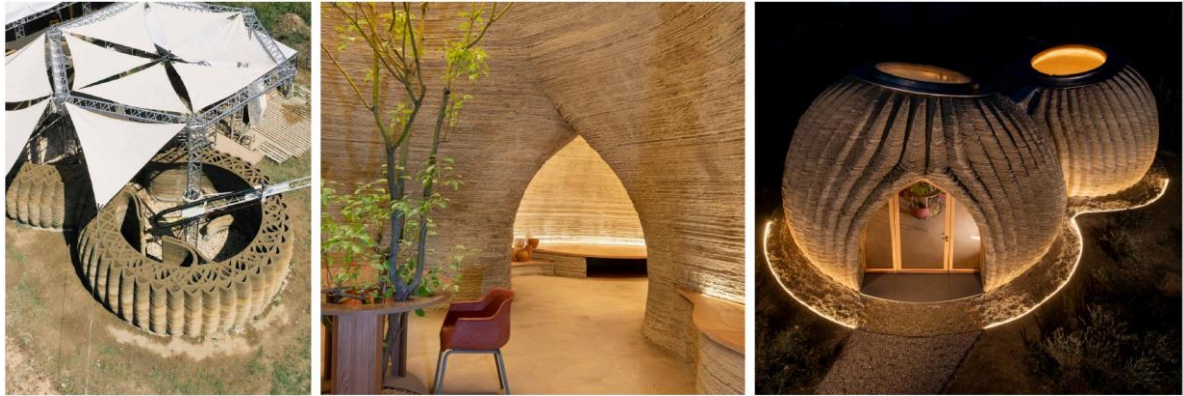
Figure 11. Images of the Tecla Project by WASP During Construction and Completed Building Source: (WASP, 2021)
