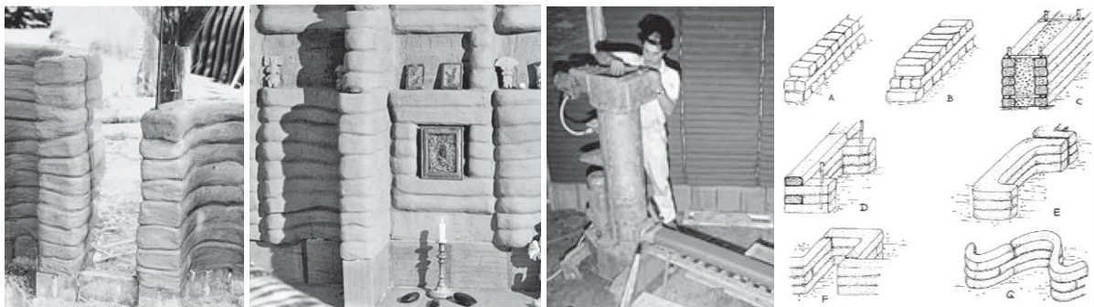
Figure 6. the Stranglehm Technique Source: (Minke, 2012)
