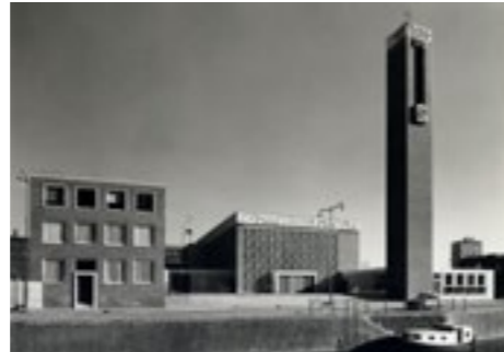
Completion of the new St. Dominic Church
