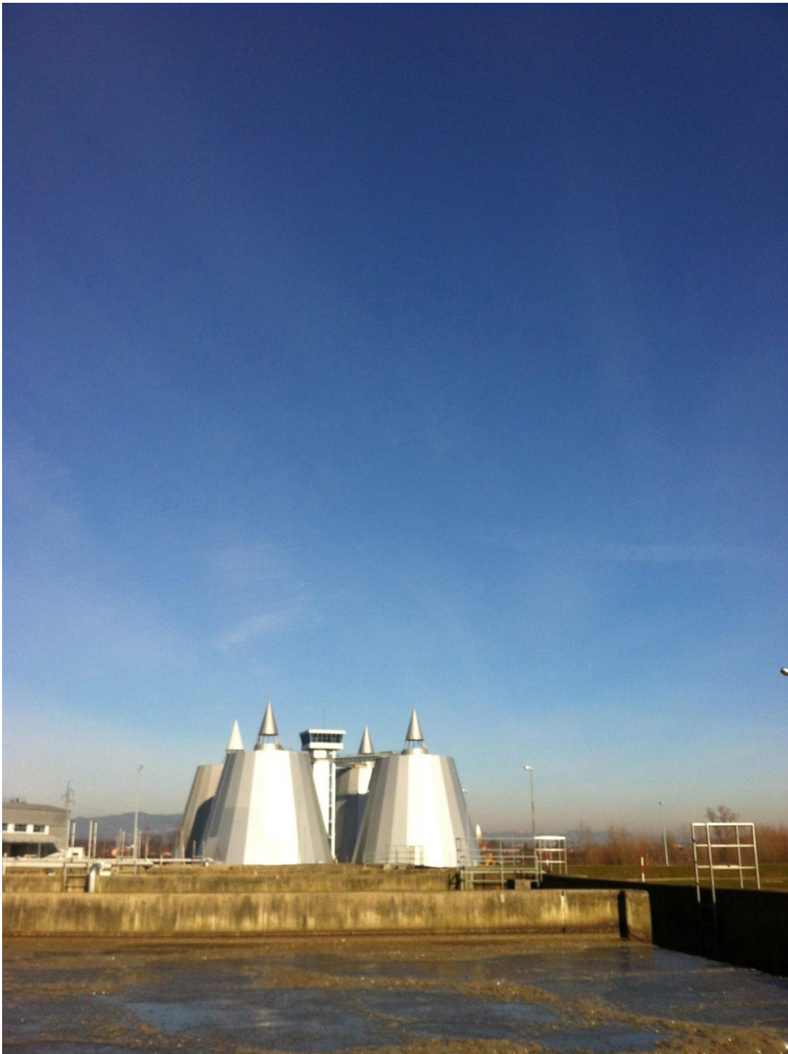
Wastewater treatment plant of city of Zagreb located in Zagreb, Croatia. The wastewater treatment plant was designed only for carbon removal. The plant was operated as a conventional activated sludge process at a solid retention time of approximately 5 days, and at an average mixed liquor suspended solids concentration of approximately 4 \text{ g L}^{-1} (Photo by Sang Yeob Kim)
