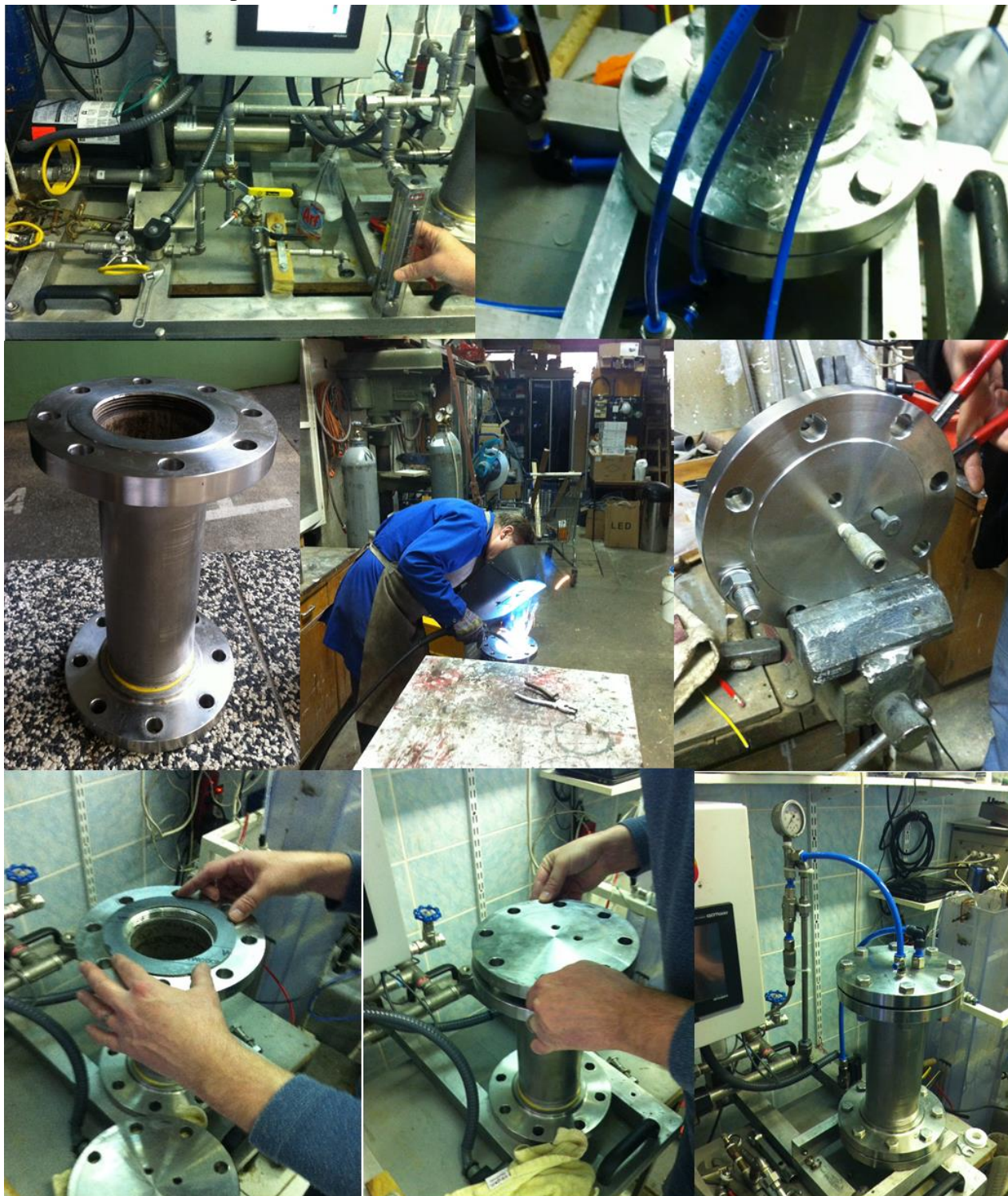
Figure 4.1 Repairing the SDOX unit
