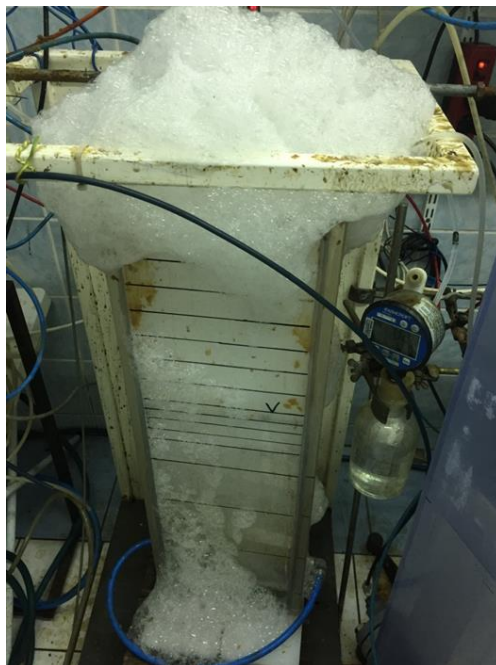
Figure 6.3 Coarse bubble diffuser cleaning
