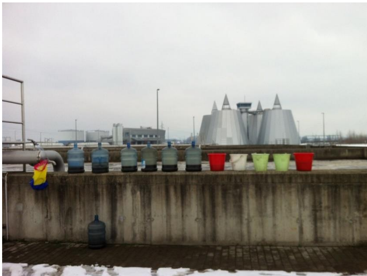
Figure 3.3 Concentrating activated sludge by gravity settling at the WWTP facility (Photo by Sang Yeob Kim)
