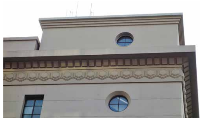
FIG. 16 Fortune Garden Kyoto, rooftop extension
