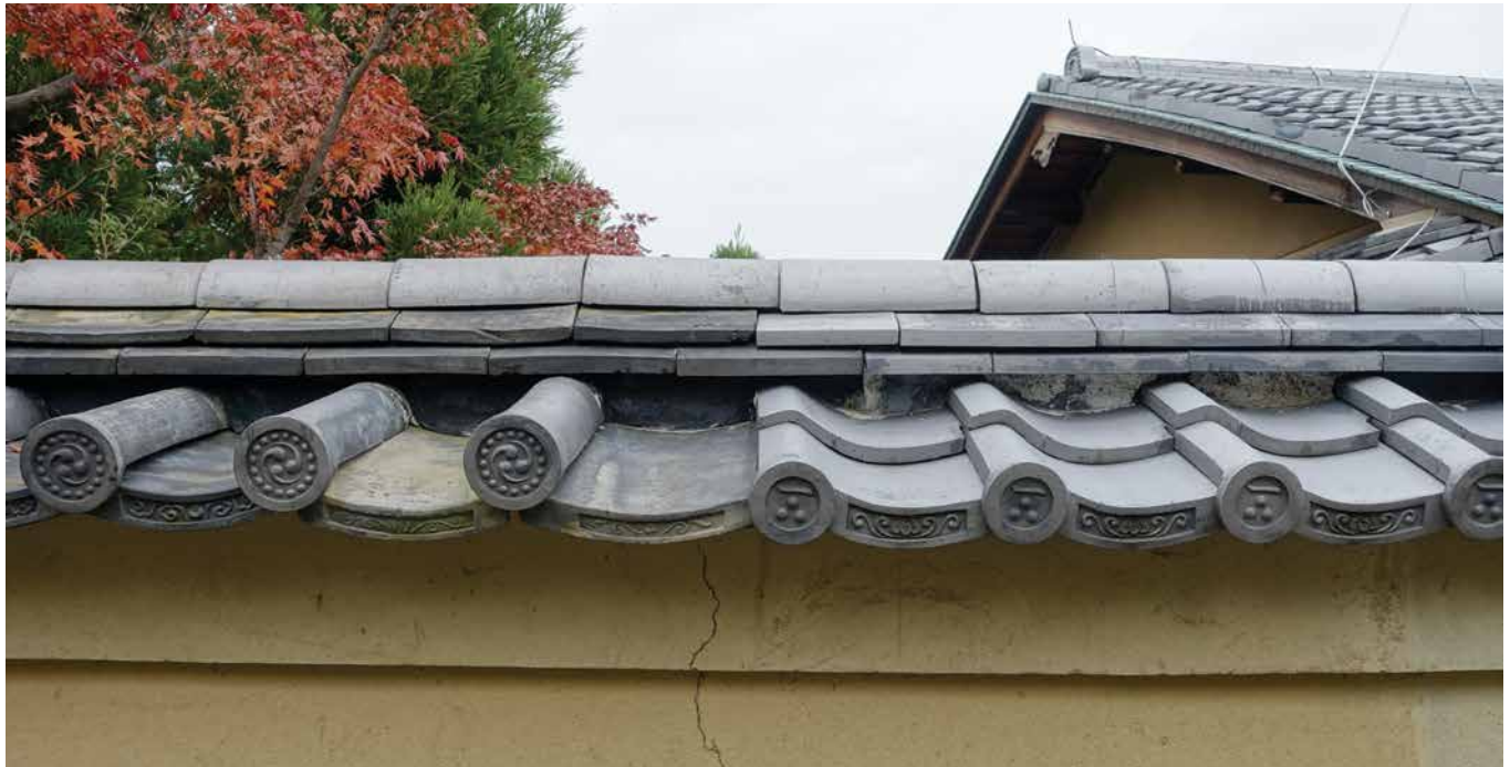
FIG. 19 Daitoku-Ji temple restored by Takamura with old and new tiles
