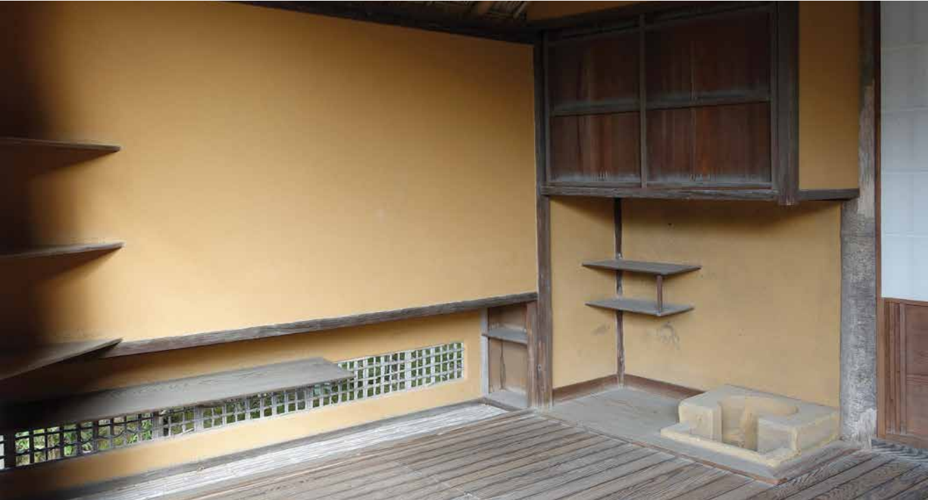
FIG. 22 Perfection in plasterwork in the buildings surrounding Katsura Imperial Villa
