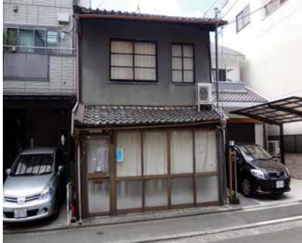
FIG. 3 Machiya before renovation
