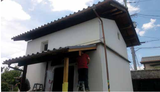
FIG. 3 Example of okabe earth wall
