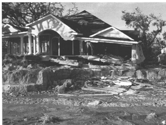
(a) Scour failure due to hurricane Katrina in 2004 (Robertson et al., 2007)
