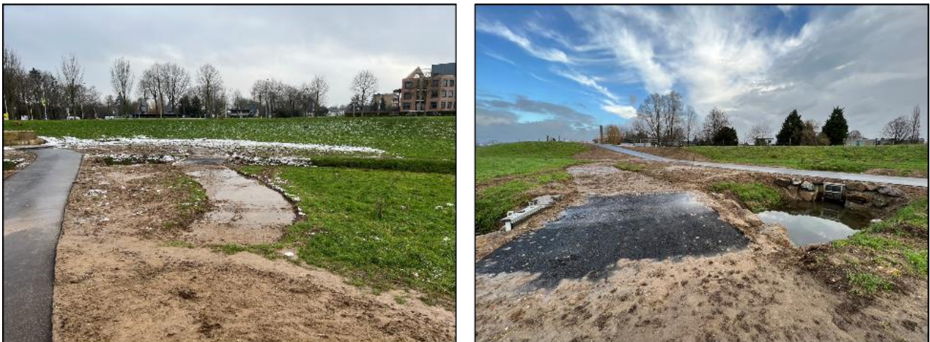
Figure 15 Actual View of the unpaved lane, scale 1:50 cm
