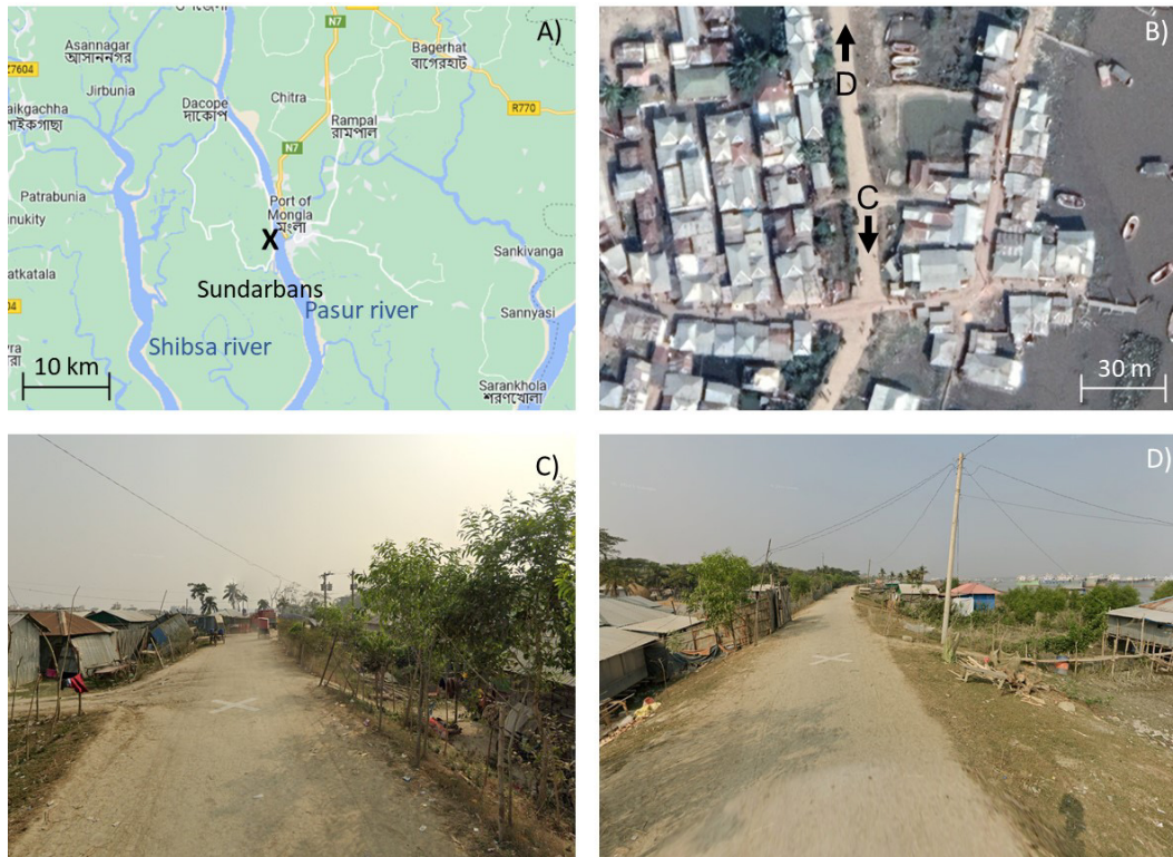
Figure 4 A) The location of the embankment site (marked by the 'X'). B) An aerial photo of the village and harbour. Letters C and D indicate the location where photos in panel C and D are taken, with arrows for their view direction. C) Photo of the embankment, with a gravel road on top and buildings on both sides. River on the left. D) Idem, with river on the right. Sources: Google Maps; Google Earth, CNES, Airbus, Maxar Technologies; Google Streetview.
