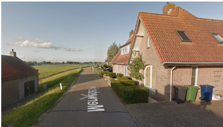
Figure 28: Location of a house at the inner slope of the embankment
