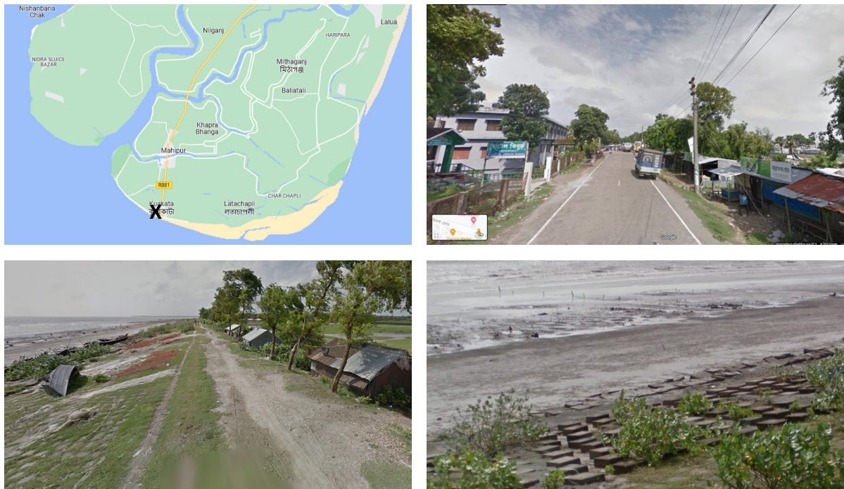
Figure 3: Photos of the sea embankment of dike ring 48. Top left: The location of the embankment site, marked by the 'X'. Top right: the embankment covered with an asphalt road, with buildings present at both inner slope (left on photo) and outer slope (right). Bottom left: some buildings present at the inner slope, stone revetment at the outer slope. Bottom right: stone revetment with roughness elements at outer slope. Sources: Google Maps, Google Streetview
