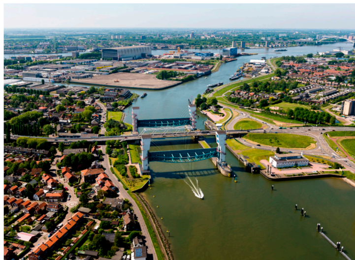
Figure 5. The Hollandse IJssel storm surge barrier as it protects the Hollandse IJssel located behind it. Courtesy Rijkswaterstaat, mediatheek.
