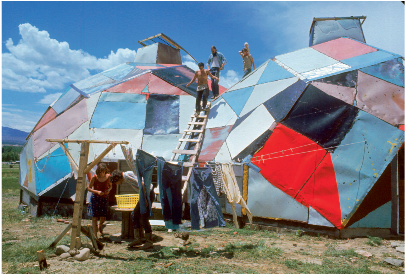
Drop City. De beplating van de koepels is afkomstig van oude auto's Drop City. Domes clad with metal sheets from disused cars.
