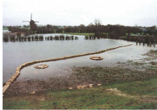
Figure 2.5: Ringed boils during high water of 1995 (TAW, 1994)
