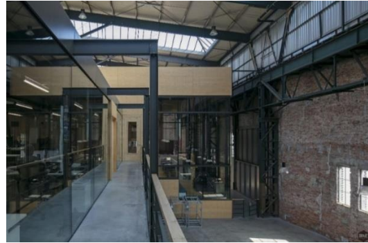
Figure 25: Similar to the imposing and recognizable structures, the built-in volume's frames are composed of steel and include gray-green profiled siding to preserve the halls ambience. The remaining infills are made of wood and glass. The use of underlayment pan
