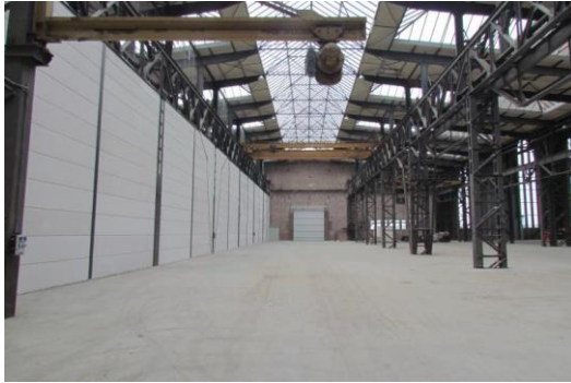
Figure 24: The hall with the partition made of unsightly material which was later installed by the Port Authority. (Adcom 2000 Architecten & Ingeneurs BV, n.d.)
