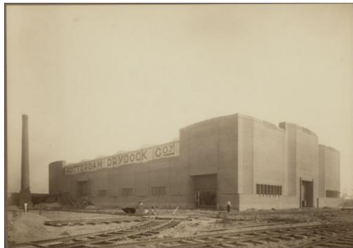
Figure 15: Exterior of the ketelmakerij . In the foreground construction of the company track. (Stadsarchief Amsterdam, 1920)
