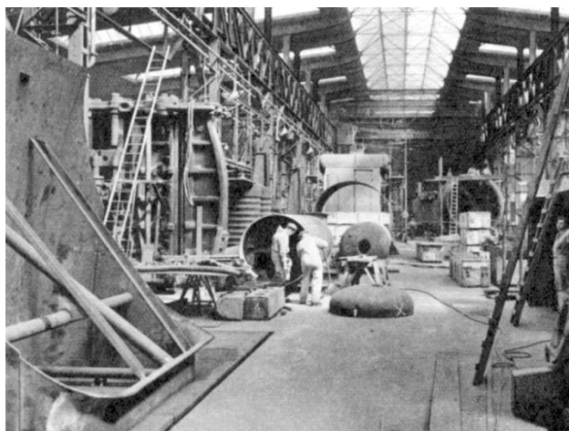
Figure 17: Work in the Ketelmakerij in 1926 (Jaarverslag RDM, 1926)
