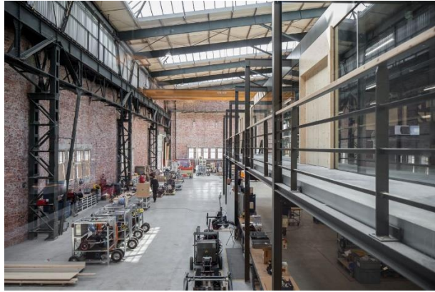
Figure 27: Completed new hall (François Verhoeven, n.d.)
