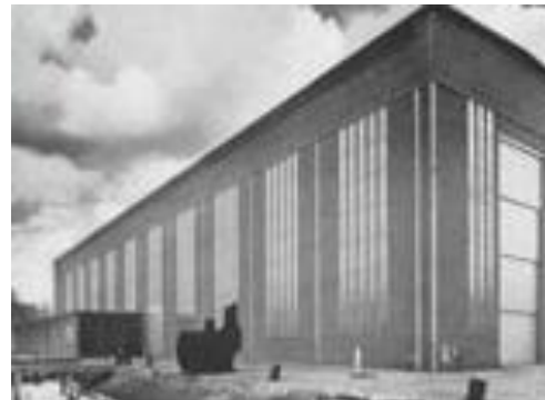
Figure 16: The 220m northern façade of the grofsmederij (Wattjes, 1940)
