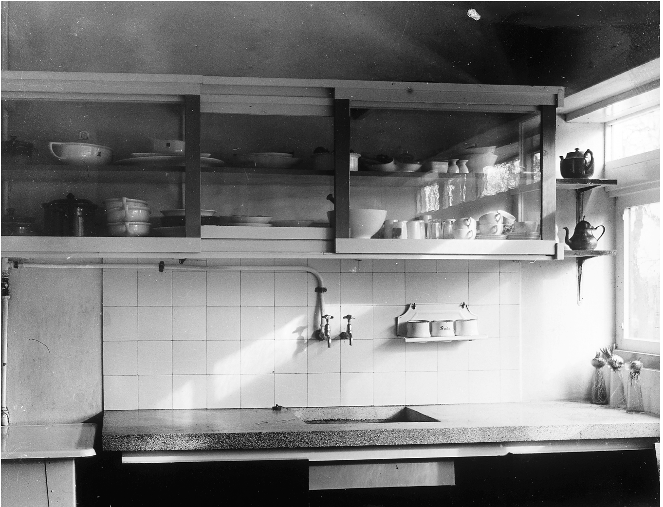
FIG. 4.44 Ground floor, kitchen, c. 1925
