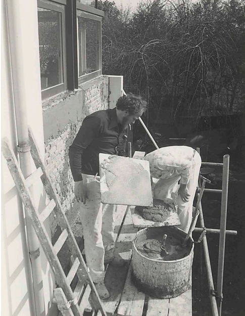
FIG. 1.10 Plasterers at work on the wall between corner window and kitchen
