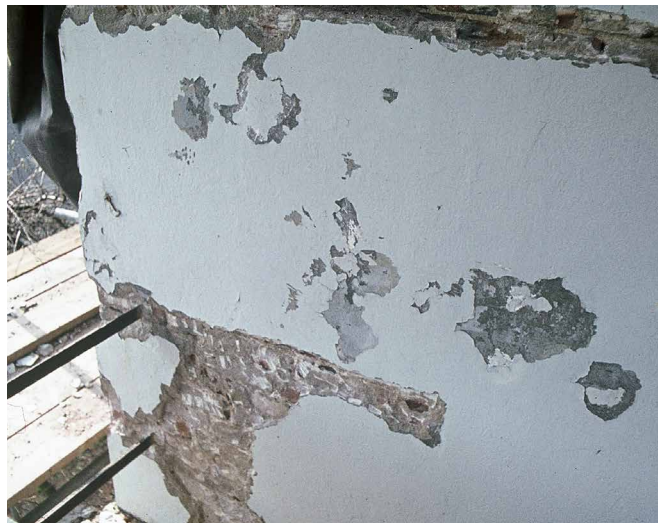
FIG. 2.7 In various places, such as the chimney, B. Mulder found still more finish coats and colours that he could include in his colour research
