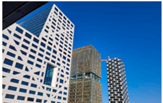
Fig. 6. Central Park building (middle) under construction (own photo, March 31, 2021).
