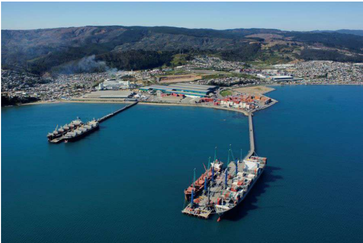
Figure B.6: Port Lirquén with mobile harbour cranes
