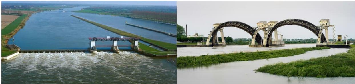
**Figure 1.** Left: Stoney-weir (2 x 17 m) and navigable Poirée-weir (63 m). Right: visor weir (2 x 48 m).
