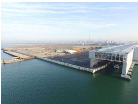
Figure 3. Reference quay structure used in the case study (Image of MUC; Alain Timmermans).
