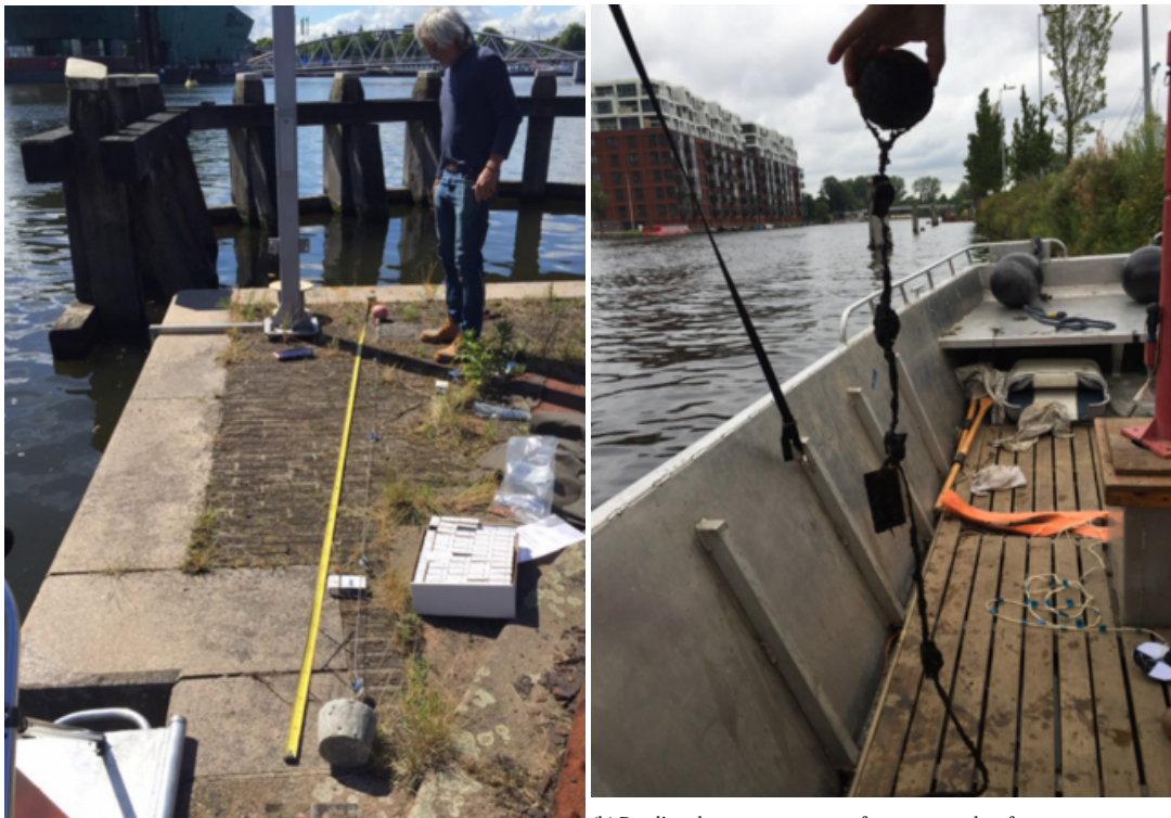
(a) Installation of the measurement equipment: the mounting of the sensors to the steel cable.
