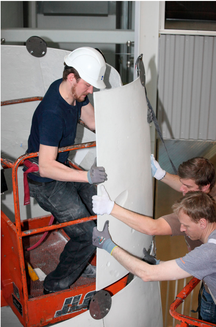
Figure 37. (a, b, c). Panel installation and final self-supporting hyperbolic shell in-situ.
