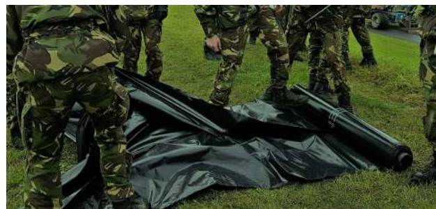
(b) Impermeable geotextile.
