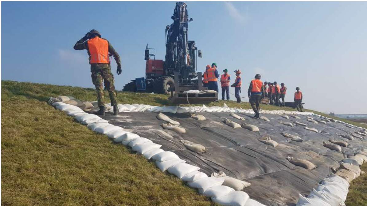
Figure F.4: Reinforcement measure Zalkerveer Zalk
