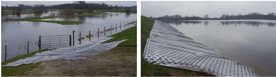
(a) Outer slope reinforcement 1.
