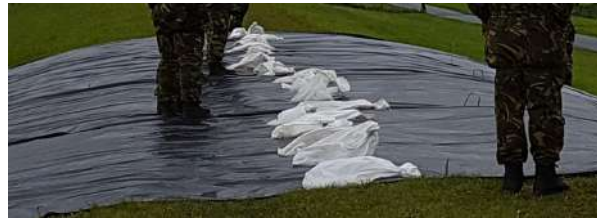
Figure 9.4: Fixation inner slope grass revetment
