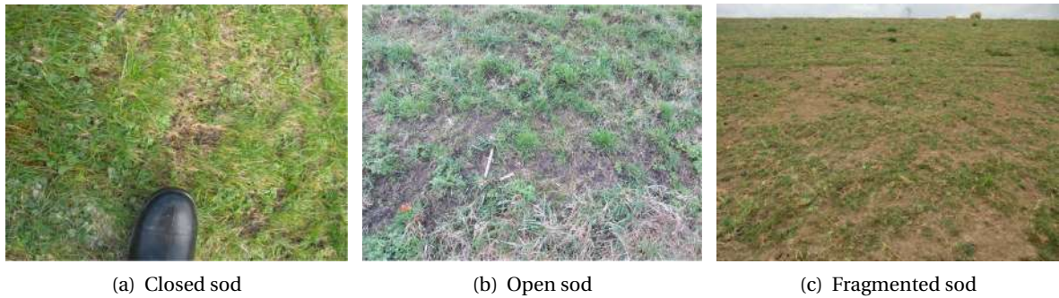
Figure A.4: Grass revetment quality (Rijkswaterstaat, 2016)
