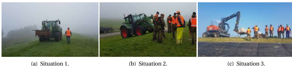
Figure 5.4: Heavy equipment on dike crest.
