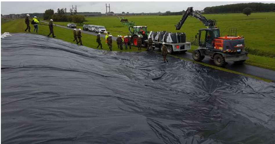
Figure C.1: Inner slope reinforcement at water board Drents Overijsselse Delta (September 16, 2017).
