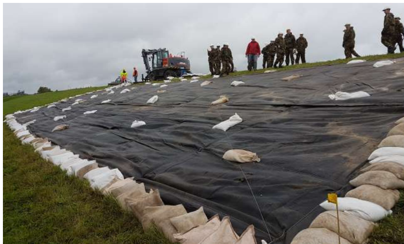
Figure F.1: Reinforcement measure Zendijk
