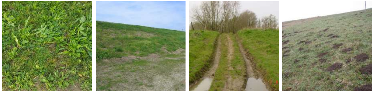
(a) Newly constructed dike Lienden (October 2017).
