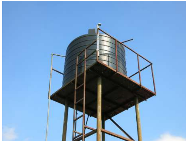
Figure 4.4: Measurement set-up at World Ahead Secondary School. The Tallysman antenna is taped to the iron structure of the watertank tower.
