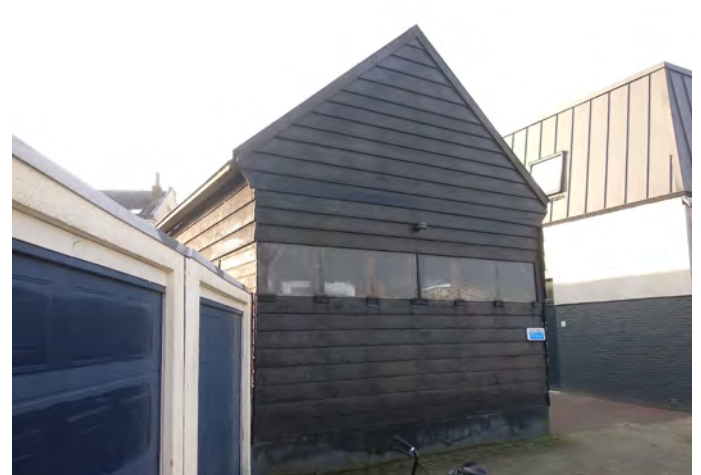
Figure 9. The carriage house in Sliedrecht. Ogees are present at the sides, just underneath the roof.
