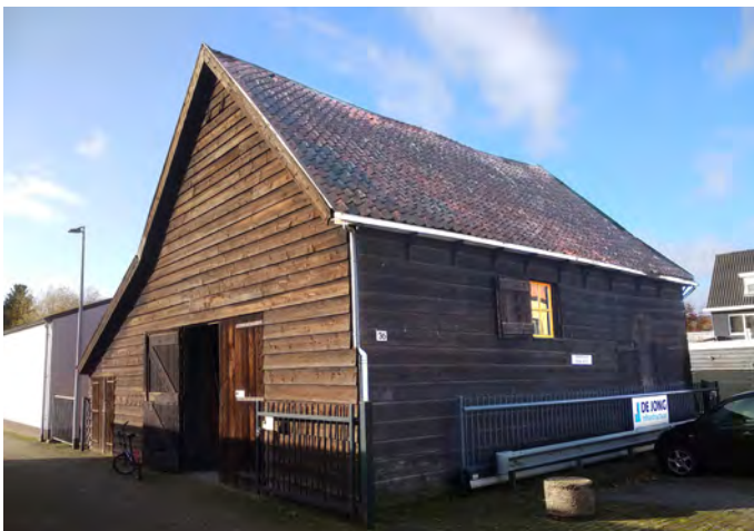
Figure 6. The northern facade, with rebated planks, and the eastern facade, with weatherboarding, of the barn in Oostendam.
