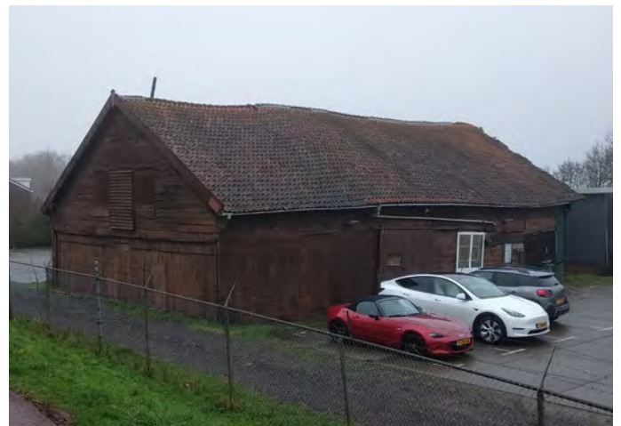
Figure 15. The southern and eastern facade of the barn in Kinderdijk.
