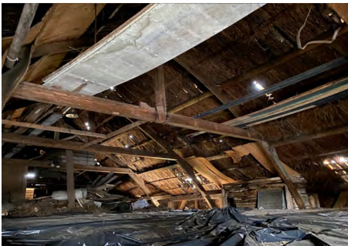
Figure 14. The Philibert trusses and the reed underneath the roof tiles of the barn in Kinderdijk. By L. de Keijzer, 2024.
