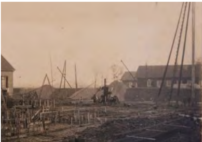
Figure 16. The western facade of the barn in Kinderdijk. From "Fotobasebank," by K. van den Heuvel, n.d. ( https://www.fotobasebank.nl/public/zoeken.php number A0064).
