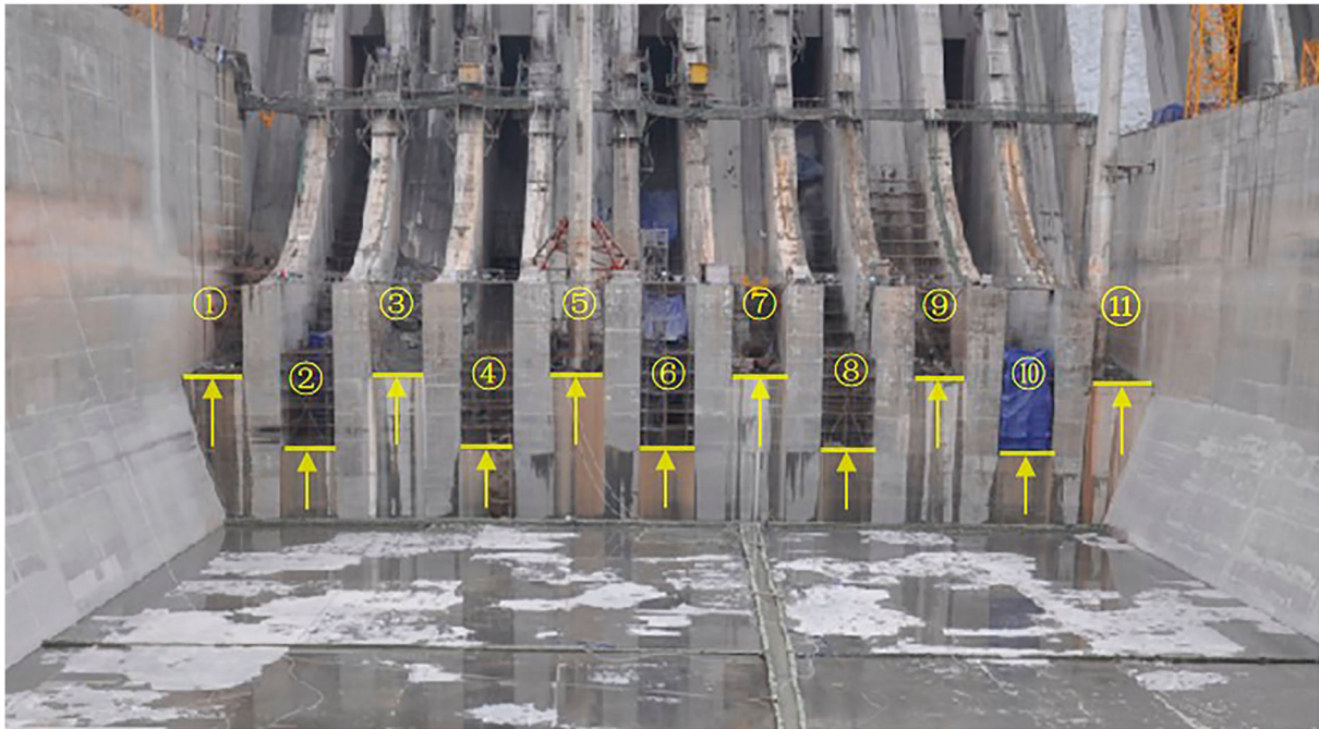
Figure 1 The Xiangjiaba Dam stilling basin with a twin-layer offset-jets inlet design, looking from downstream. The 11 spillway outlets are numbered from ① to ⑪ and the negative step edges remarked with arrows. Courtesy of Zhipan Niu. Chen et al. (2014) reported higher energy dissipation rates for a similar design based on physical modelling compared to classic hydraulic jumps and spatial B-jumps
