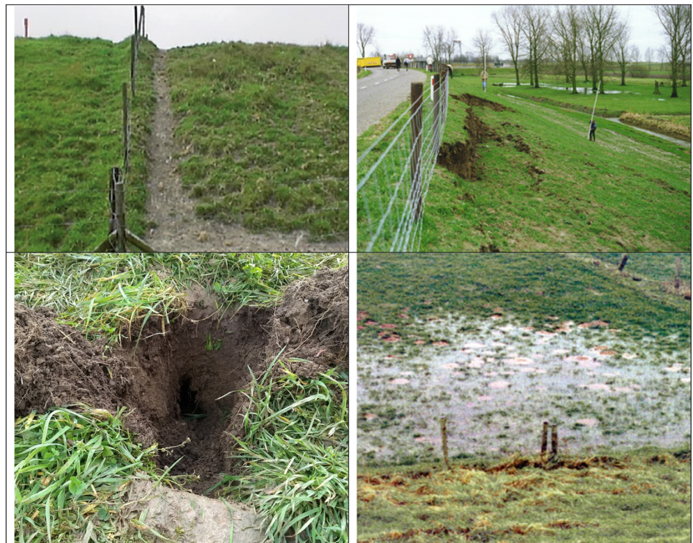
FIGURE 3 Examples of performance indicators. Local subsidence due to trampling by livestock (upper left; picture from STOWA, 2018), severe subsidence (upper right; picture from STOWA, 2018), animal burrowing (lower left, picture taken by S.J.H.Rikkert, 2020), and wet spots at the levee toe (lower right; picture from STOWA, 2018)
