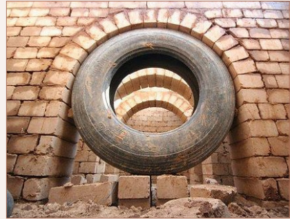
Figure 11.16 Car-Tire Used as a Formwork
