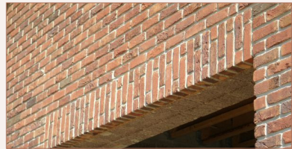
Figure 11.17 Rectangular Window / Door Opening
