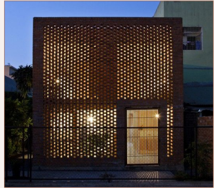
Figure 11.18 Perforated Brickwork at Reference Project Termitary House, Vietnam
