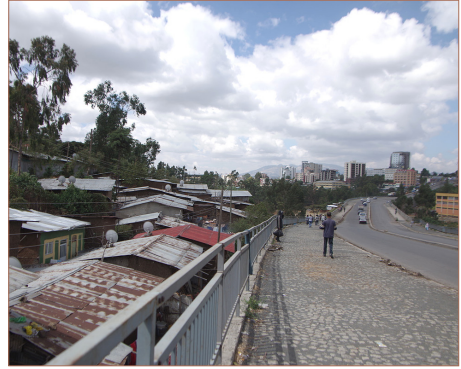
Figure 3.6 View on the Rwanda Street at the site's entrance [Source: Google Earth ]
