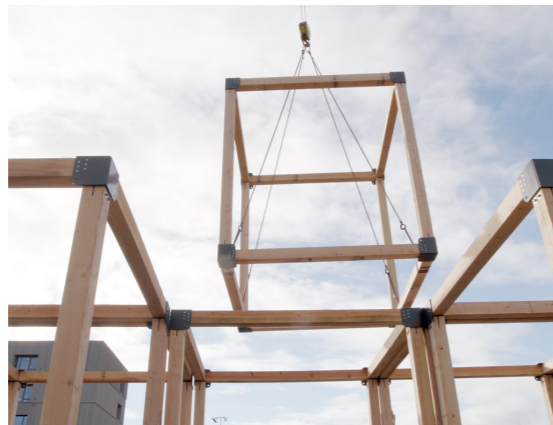
The Natural Pavillion, 2022
